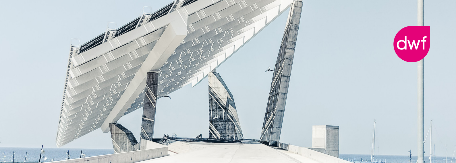
Forum Photovoltaic Power Plant, Barcelona
